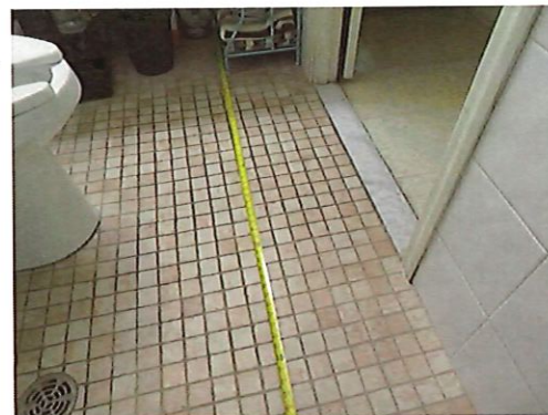
UFAS Unit 22 Two Bedroom One Bathroom (occupied): Bathroom Width
