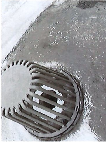
77. Typical Roof Drain
