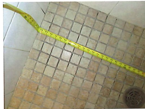
UFAS Unit 22 Two Bedroom One Bathroom (occupied): Shower Width
