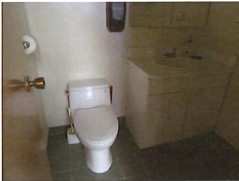
Leasing Office Restroom
