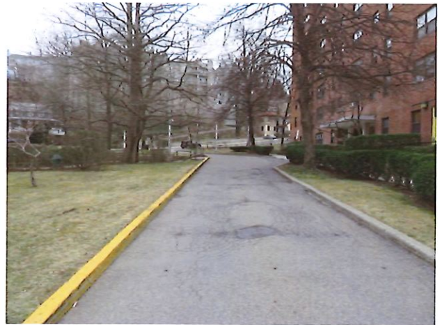
34. Property Entrance Facing Franklin Street
