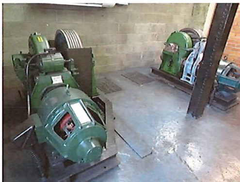
Elevator Brakes/Machinery
