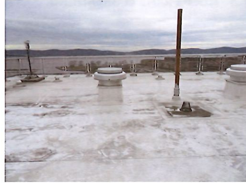
View of Roof
