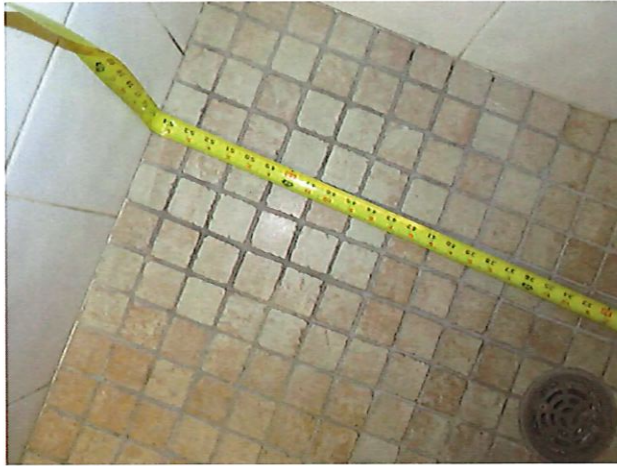
65. UFAS Unit 22 Two Bedroom One Bathroom (occupied): Shower Width
