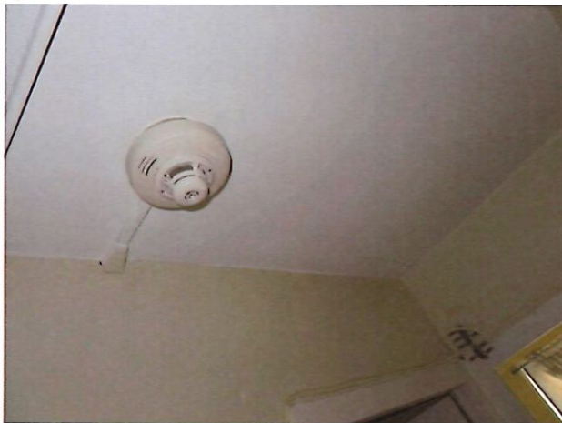
39. Unit 91 Three Bedroom One Bathroom (occupied): Typical Smoke Alarm
