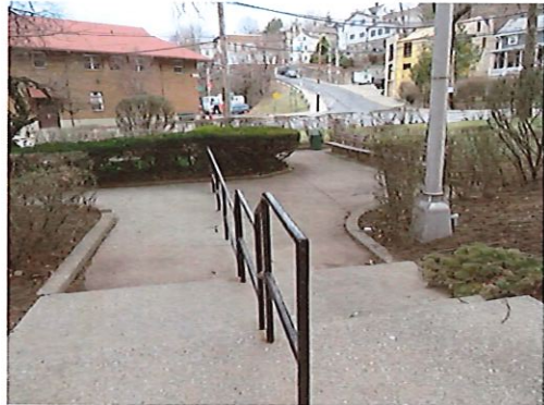
Outdoor Steps and Metal Handrail
