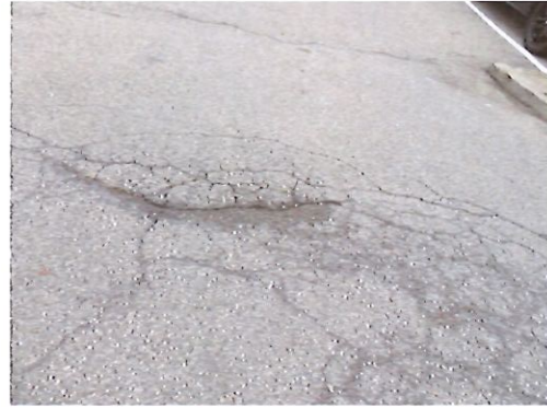
Pothole Repair for Asphalt Parking Lot (Non-Critical Repair)
