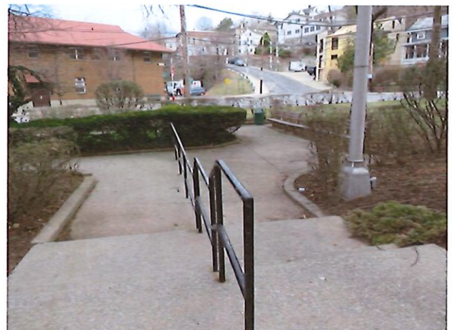
36. Outdoor Steps and Metal Handrail
