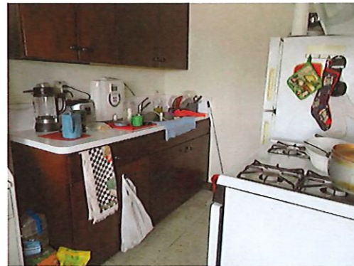
Unit 88 One Bedroom One Bathroom (occupied): Kitchen
