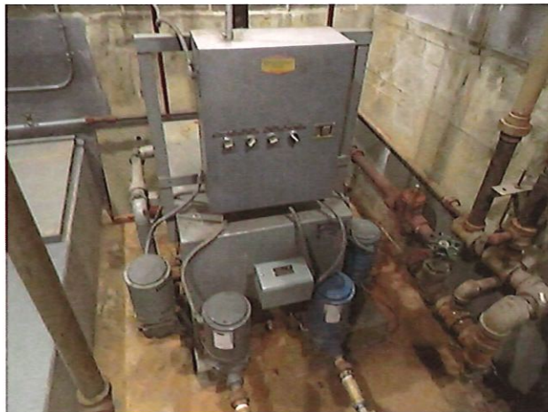
87. Vacuum Heating Pump
