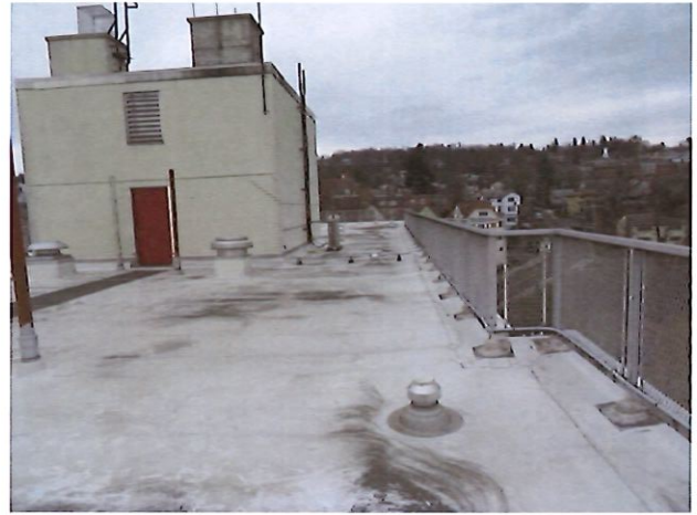
74. View of Exterior Elevator Maintenance Room
