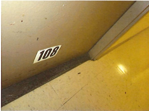
29. Unit 108 One Bedroom One Bathroom (occupied): Front Door
