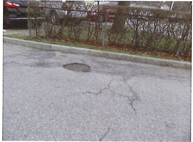
26. Pothole Repair for Asphalt Parking Lot (Non-Critical Repair)
