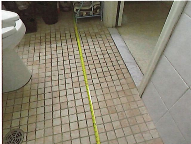
67. UFAS Unit 22 Two Bedroom One Bathroom (occupied): Bathroom Width
