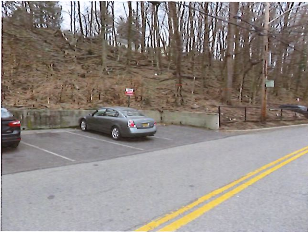
33. Retaining Wall and Parking Along Franklin Court
