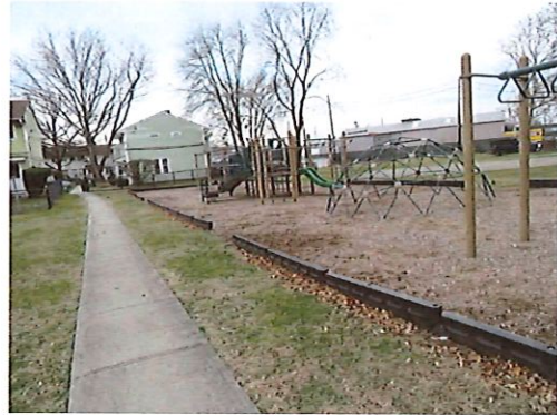
Concrete Sidewalk Near Playground
