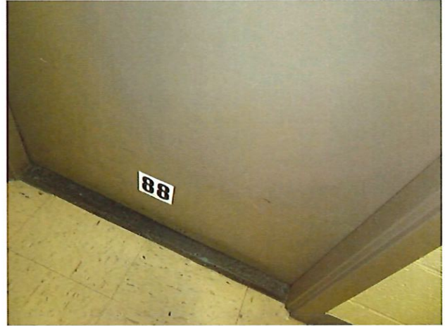
50. Unit 88 One Bedroom One Bathroom (occupied): Front Door
