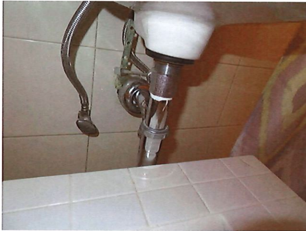
17. UFAS Unit 103 Two Bedroom One Bathroom (occupied): Bathroom Sink Needs Scald and Abrasion (Critical Repair)
