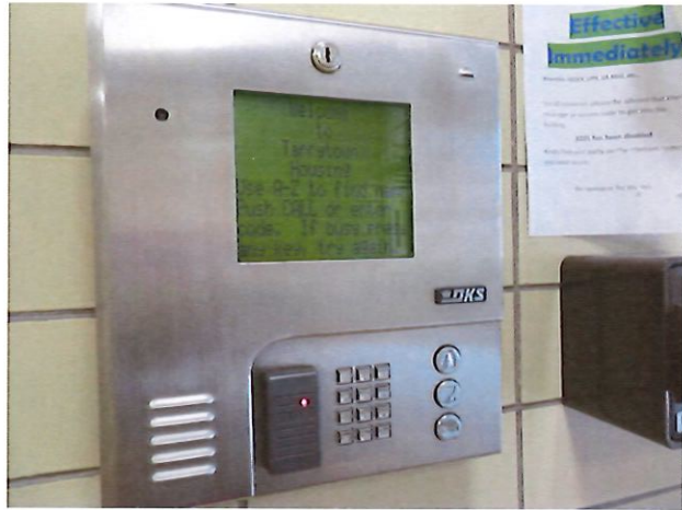
9. Buzzer Intercom System
