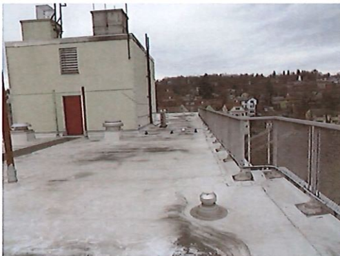
View of Exterior Elevator Maintenance Room
