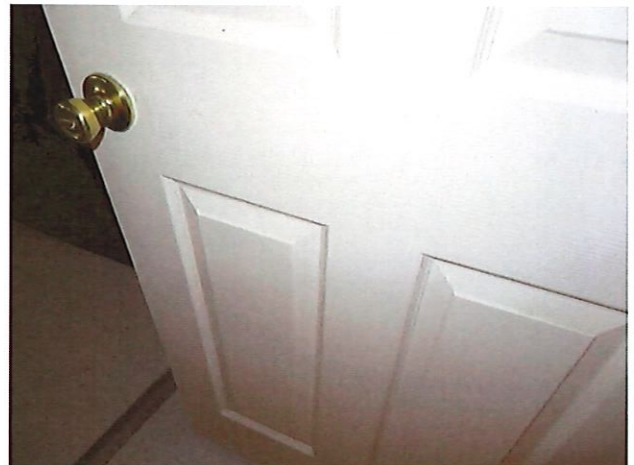
12. UFAS Unit 103 Two Bedroom One Bathroom (occupied): Bathroom Door Doesn't Have Levered Hardware (Critical Repair)
