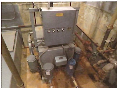
Vacuum Heating Pump
