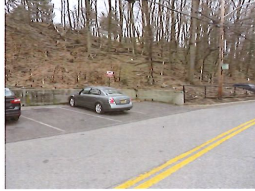
Retaining Wall and Parking Along Franklin Court
