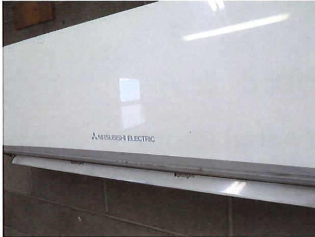
85. Indoor Split-System Heat Pump
