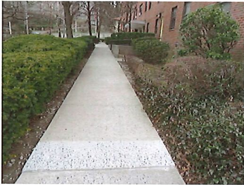
Concrete Sidewalk Near Leasing Office
