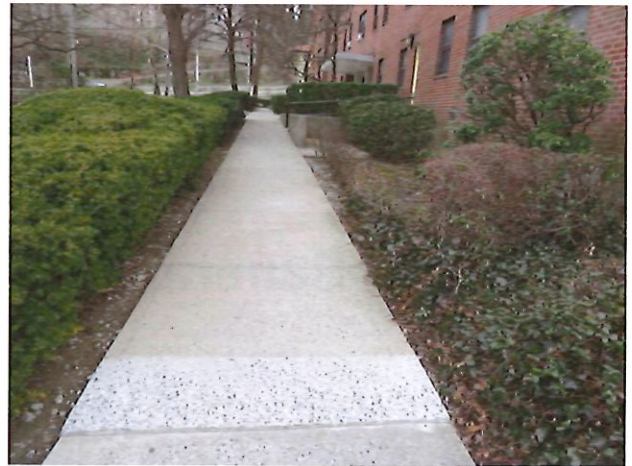
2. Concrete Sidewalk Near Leasing Office
