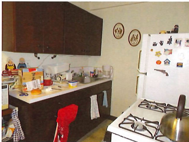
31. Unit 108 One Bedroom One Bathroom (occupied): Kitchen
