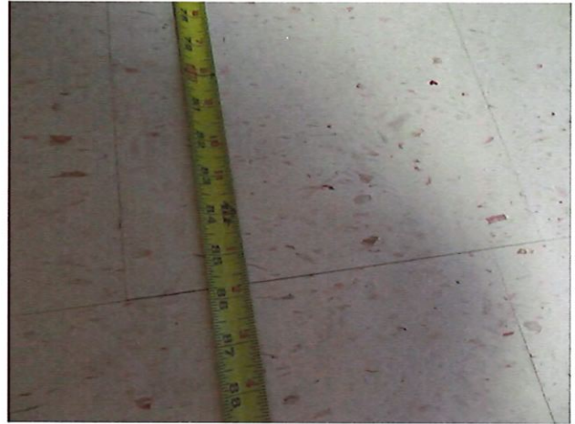
10. UFAS Unit 103 Two Bedroom One Bathroom (occupied): Kitchen Width
