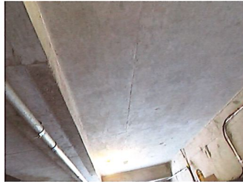
Lightweight Concrete Ceiling
