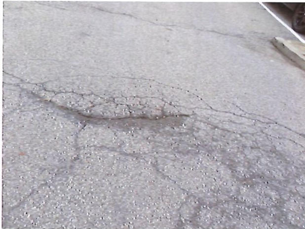
27. Pothole Repair for Asphalt Parking Lot (Non-Critical Repair)
