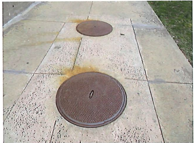
40. Storm Drain Manhole
