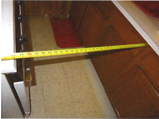
69. UFAS Unit 22 Two Bedroom One Bathroom (occupied): Kitchen Distance Between Cabinets
