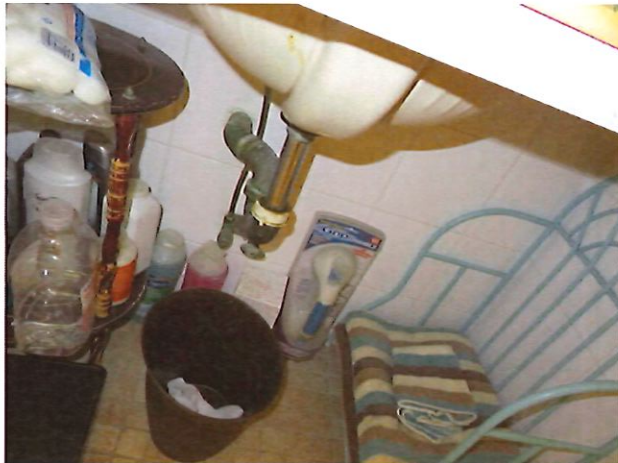
63. UFAS Unit 22 Two Bedroom One Bathroom (occupied): Bathroom Sink No Scald and Abrasion (Critical Repair)
