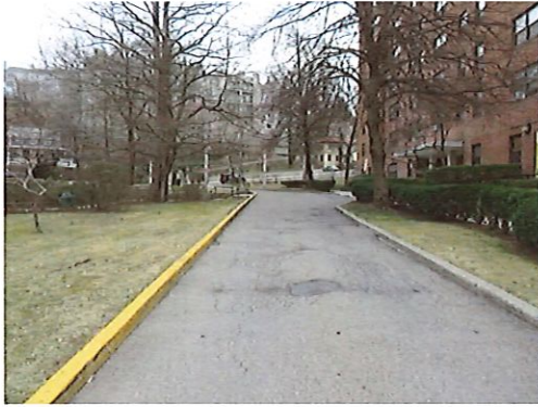
Property Entrance Facing Franklin Street
