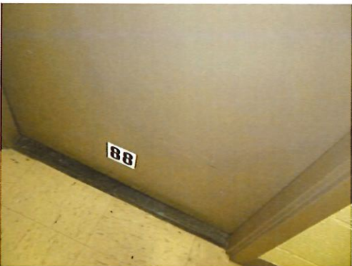
Unit 88 One Bedroom One Bathroom (occupied): Front Door
