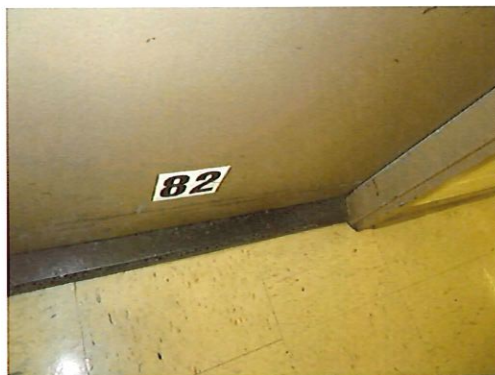
Unit 82 Two Bedroom One Bathroom (occupied): Front Door
