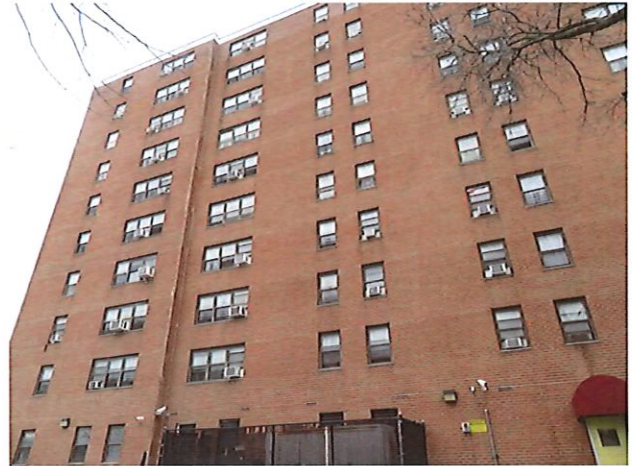
62. Exterior Backside View of Building
