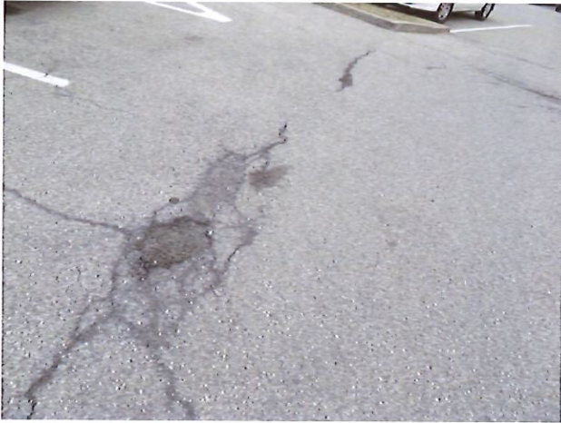
25. Pothole Repair for Asphalt Parking Lot (Non-Critical Repair)
