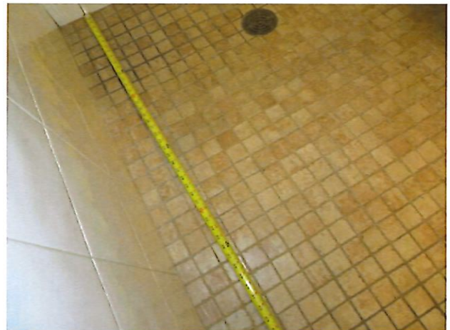
64. UFAS Unit 22 Two Bedroom One Bathroom (occupied): Shower Length
