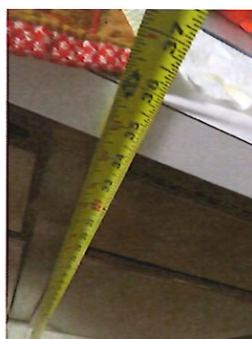
UFAS Unit 103 Two Bedroom One Bathroom (occupied): Kitchen Sink Height
