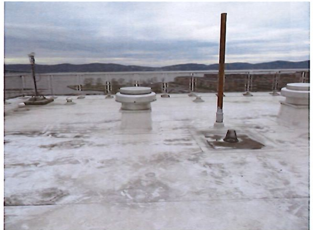
76. View of Roof
