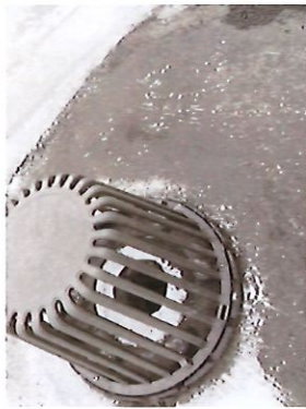
Typical Roof Drain
