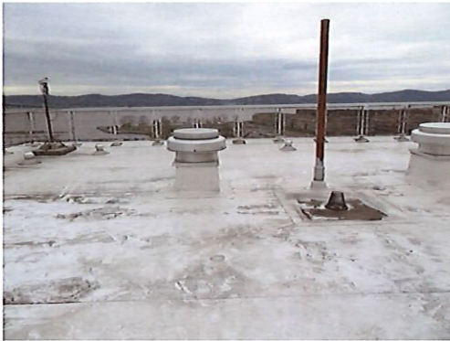
View of Roof
