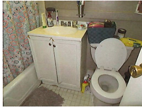
Unit 82 Two Bedroom One Bathroom (occupied): Bathroom
