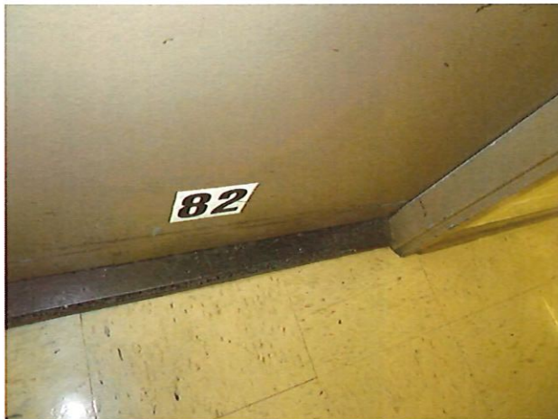
43. Unit 82 Two Bedroom One Bathroom (occupied): Front Door
