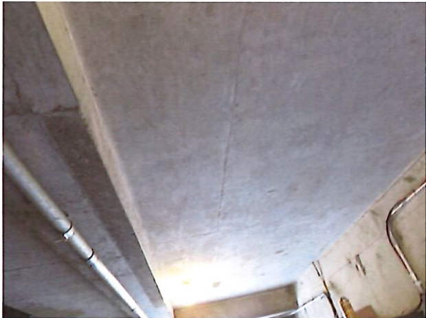
75. Lightweight Concrete Ceiling
