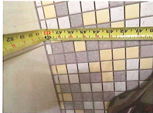
UFAS Unit 103 Two Bedroom One Bathroom (occupied): Bathroom Width
