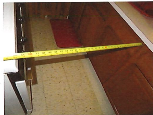
UFAS Unit 22 Two Bedroom One Bathroom (occupied): Kitchen Distance Between Cabinets
